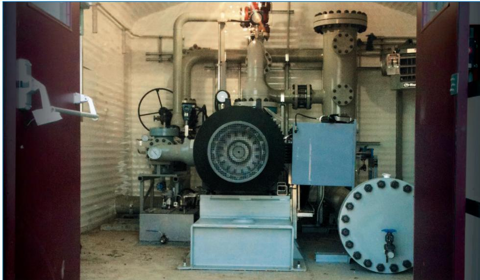
The Leistritz Multiphase Wellhead System (MWS) is a proven and economical method of artificial lift that accelerates production by lowering wellhead pressure and/or boosting discharge pressure to buck pipeline pressure. MWSs handle total flow rates up to 100,000
