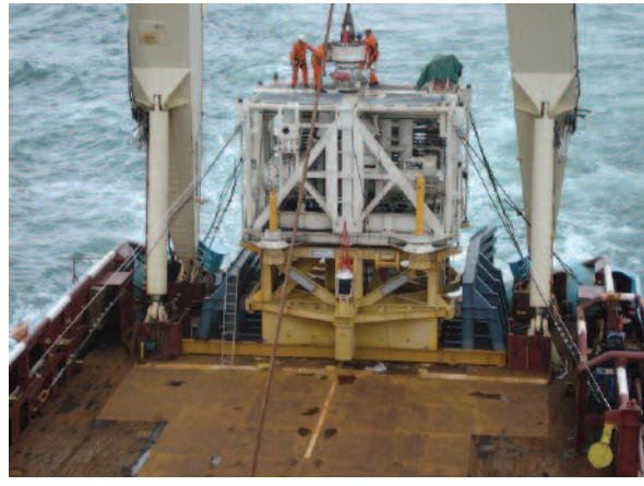
Subsea boosting is emerging as a major growth area for multiphase pumping, and is a key driver for future advancements in multiphase technology. A sharp rise is expected in subsea multiphase boosting installations in deep- and ultra-deepwater fields, some of which cannot be produced without boosting from the first day of production. This photo shows a pump as it is being prepared for deployment in subsea service.
